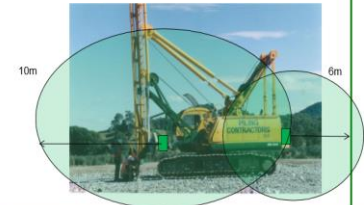
Safe zone working
